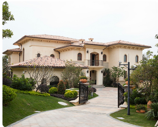
Access to the compound
