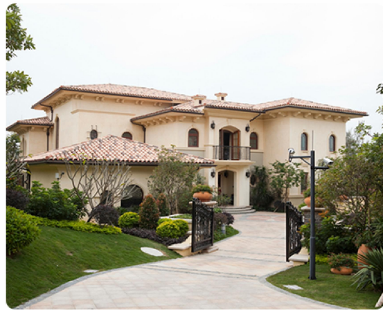
Access to the compound
